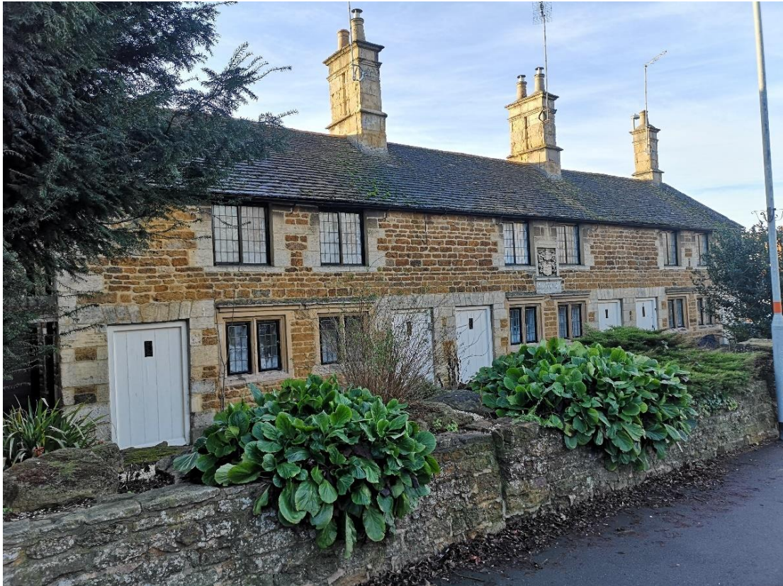
Sawyer's Almshouses, Sheep Street, Kettering
